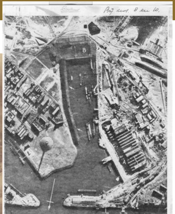
E/R BOAT SHELTERS AT IJMUIDEN. A second concrete shelter (A) under construction at the E. R. boog base at IJmuiden, as it appeared on January 30th. Like the existing shelter (B), it has a series of parallel bays and is equipped with workshops. In front of the shelter is a temporary dam which will be removed on completion. On the east side of the Herring Harbour a net awning (arrows) has been erected, presumably to hide vessels when they are in the base. Bad weather will usually cause this type of camouflage to disintegrate in time. Note how the existing concrete shelter has been camouflaged by netting stretched from the roof to the ground.
